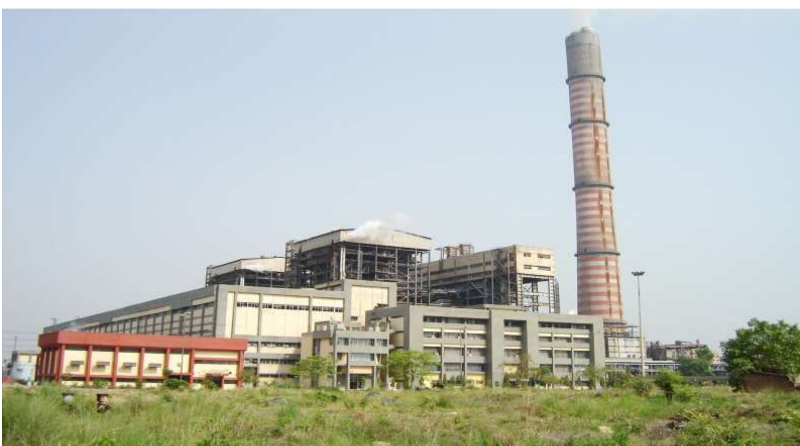
Picture 1: Tenughat Vidyut Nigam Limited (TVNL) 2*210 MW Power Plant
